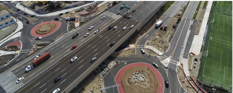
Alameda CTC investments in projects like the I-80 Gilman Interchange Improvement Project advance safety, strengthen interstate connections and support the movement of people and goods throughout the region.
