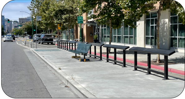
Upgraded Bus Stops and Rider Waiting Areas
