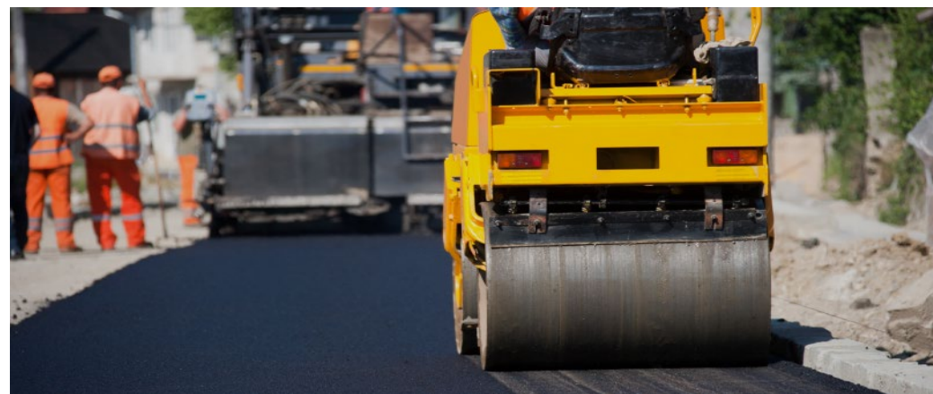
City of Hayward – Street Rehabilitation
