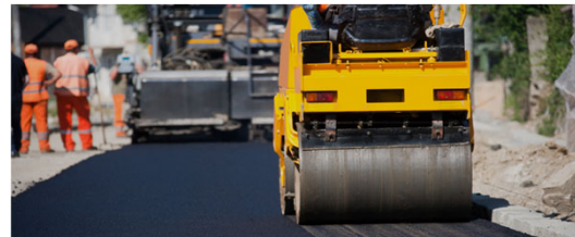
City of Hayward – Street Rehabilitation
