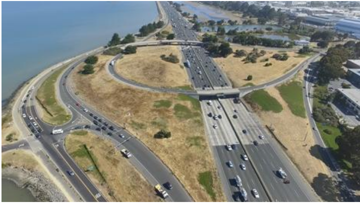
Aerial view of I-80/Ashby Avenue (SR-13) interchange.
