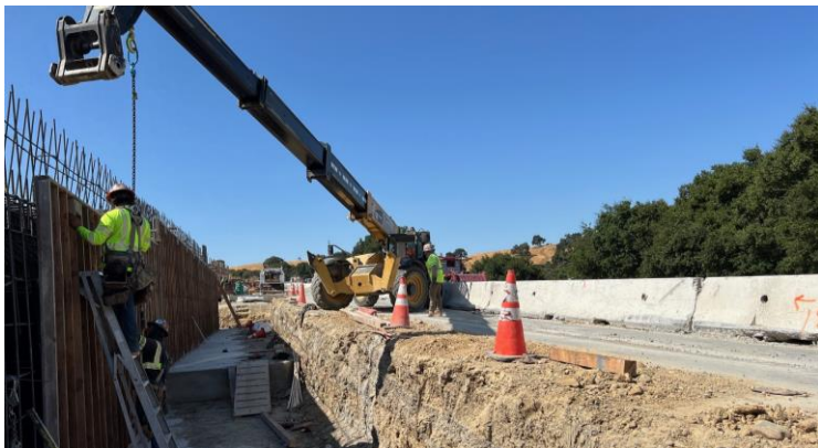
Work on the new I-680 median north of Koopman Bridge.
