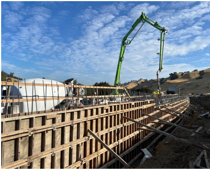
Work on the new I-680 median.
