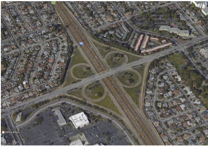
Current interchange at I-880/Winton Avenue.
