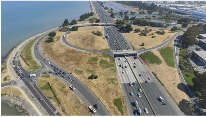
Aerial view of I-80/Ashby Avenue (SR-13) interchange.
