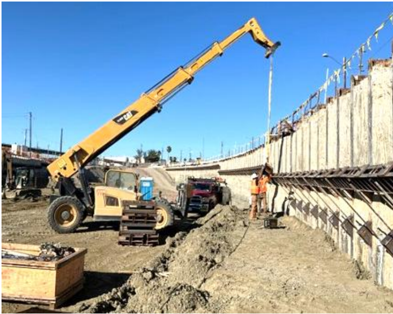
Reinforcement being added to allow for excavation of new underpass.
