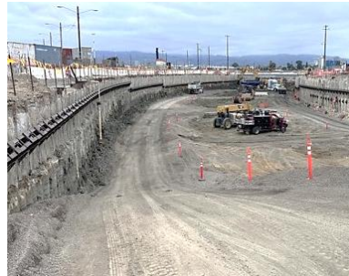
Excavation for the new 7th Street on west end of project.
