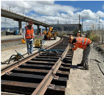
New UPRR railway track being constructed on new alignment.
