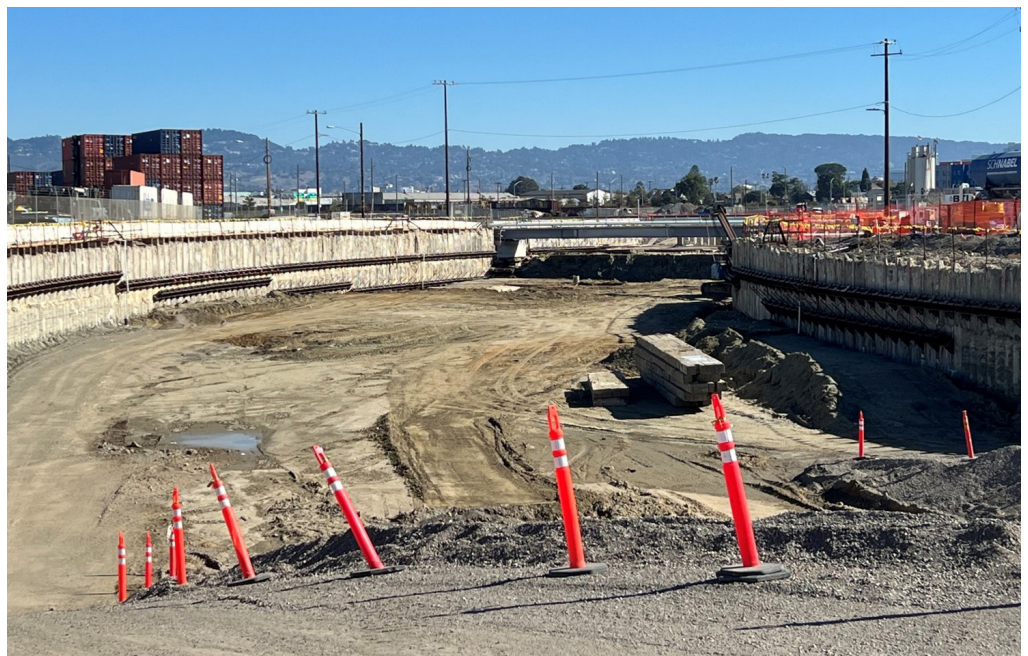
New 7th St. Grade Separation East alignment – looking east. Picture shows roadway excavation area, deep soil mix and tie-back wall installations.
