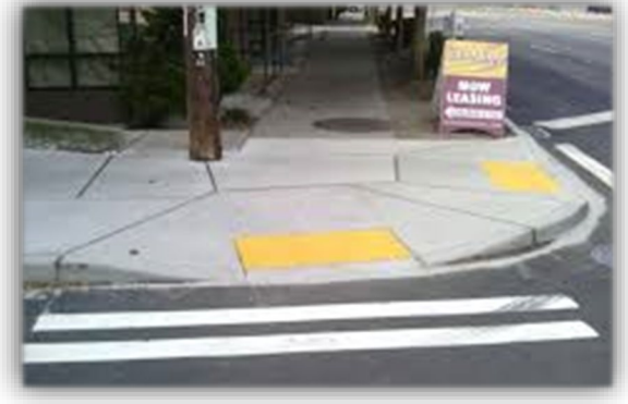
Accessible curb ramps
