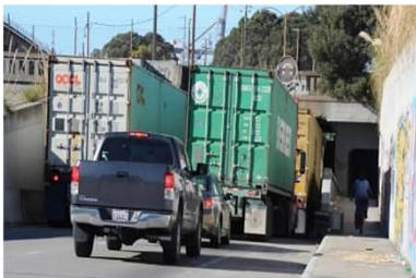
Truck stuck at the 7th Street underpass.
