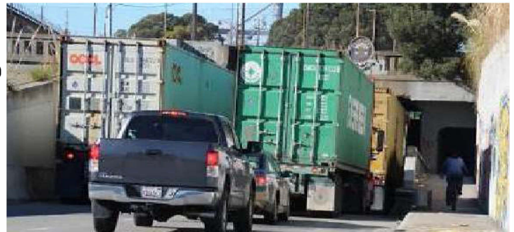
Existing 7th Street underpass with low clearance and lane width
