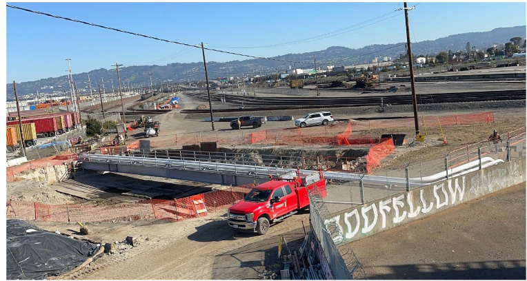
New Kinder Morgan Pipelines on New Bridge Jan 2025
