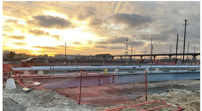
New Kinder Morgan bridge is set.
