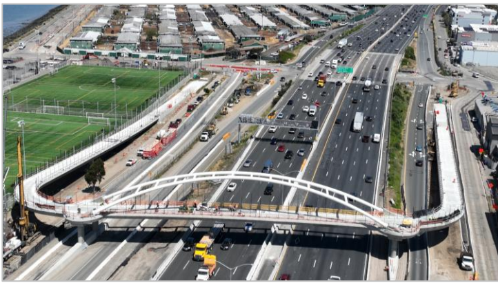
Bicycle and pedestrian overcrossing that is Phase 1 of the I-80 Gilman Interchange Improvements project.
