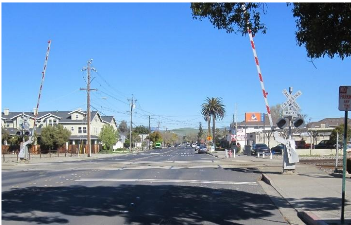
Rail crossing on L Street in the City of Livermore.
