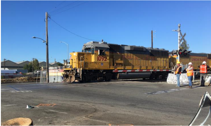
Rail crossing along 37th Avenue in the City of Oakland.
