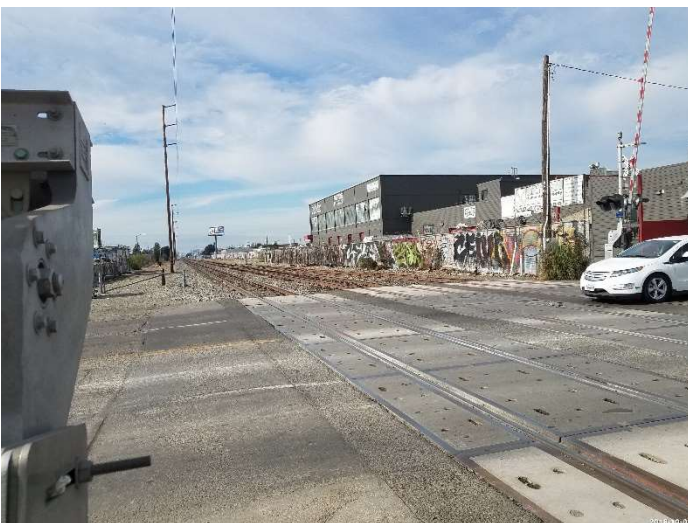
Railroad Right-of-Way, West Facing
