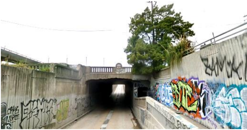
7th Street, approaching Union Pacific Railroad bridge from the east.
