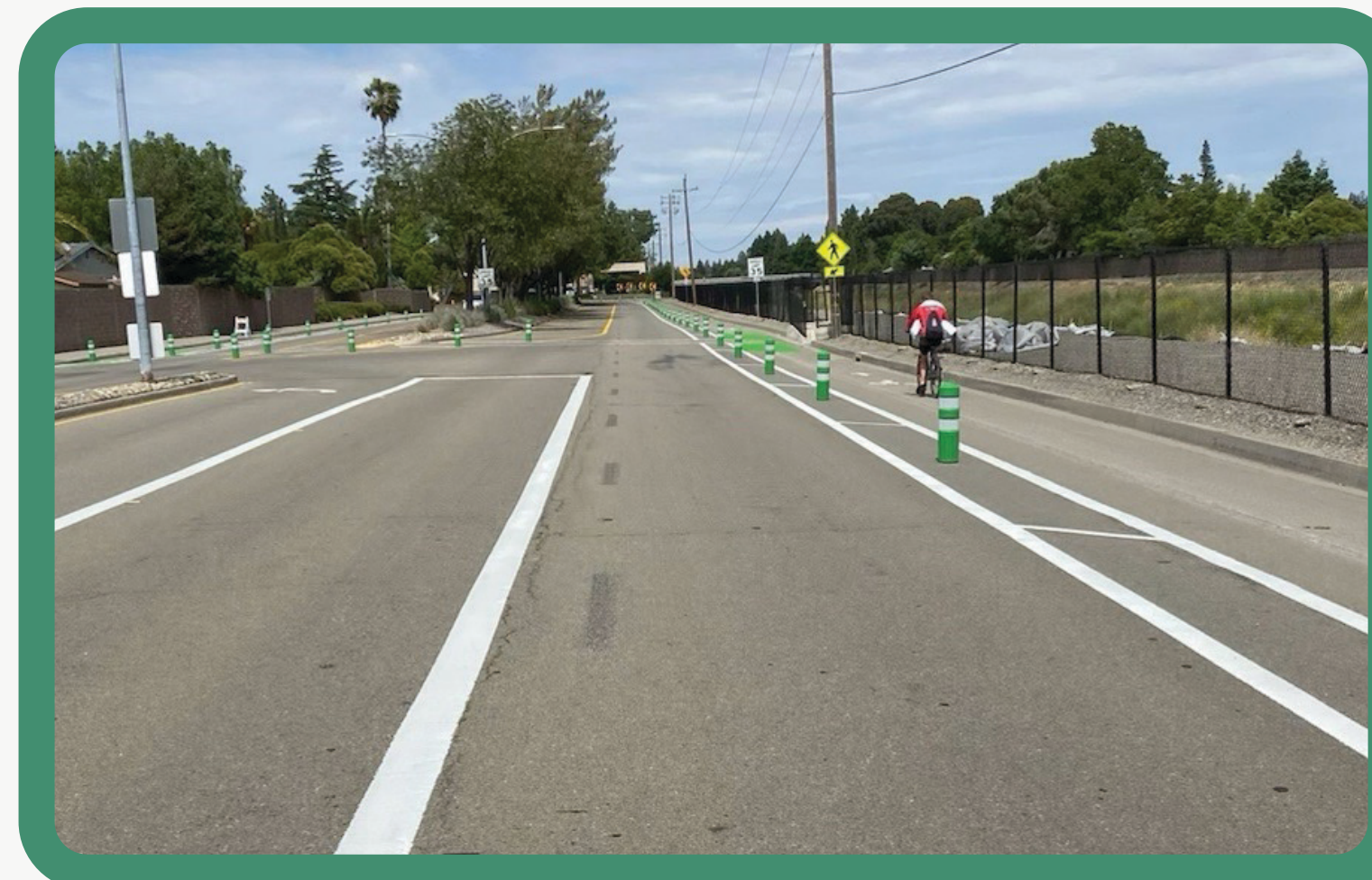
Quick Build Protected Bike Lane
