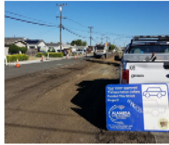
City of San Leandro – Street Rehabilitation (Corvallis St.)
