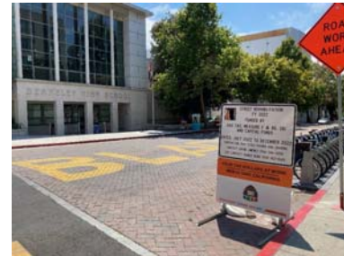
City of Berkeley – Pavement Rehabilitation Program (Milvia St.)
