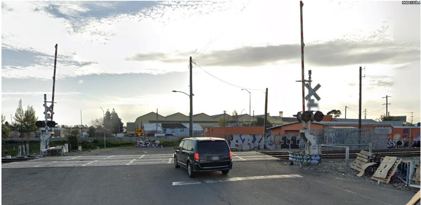
Figure 4: 37 th Avenue Crossing
