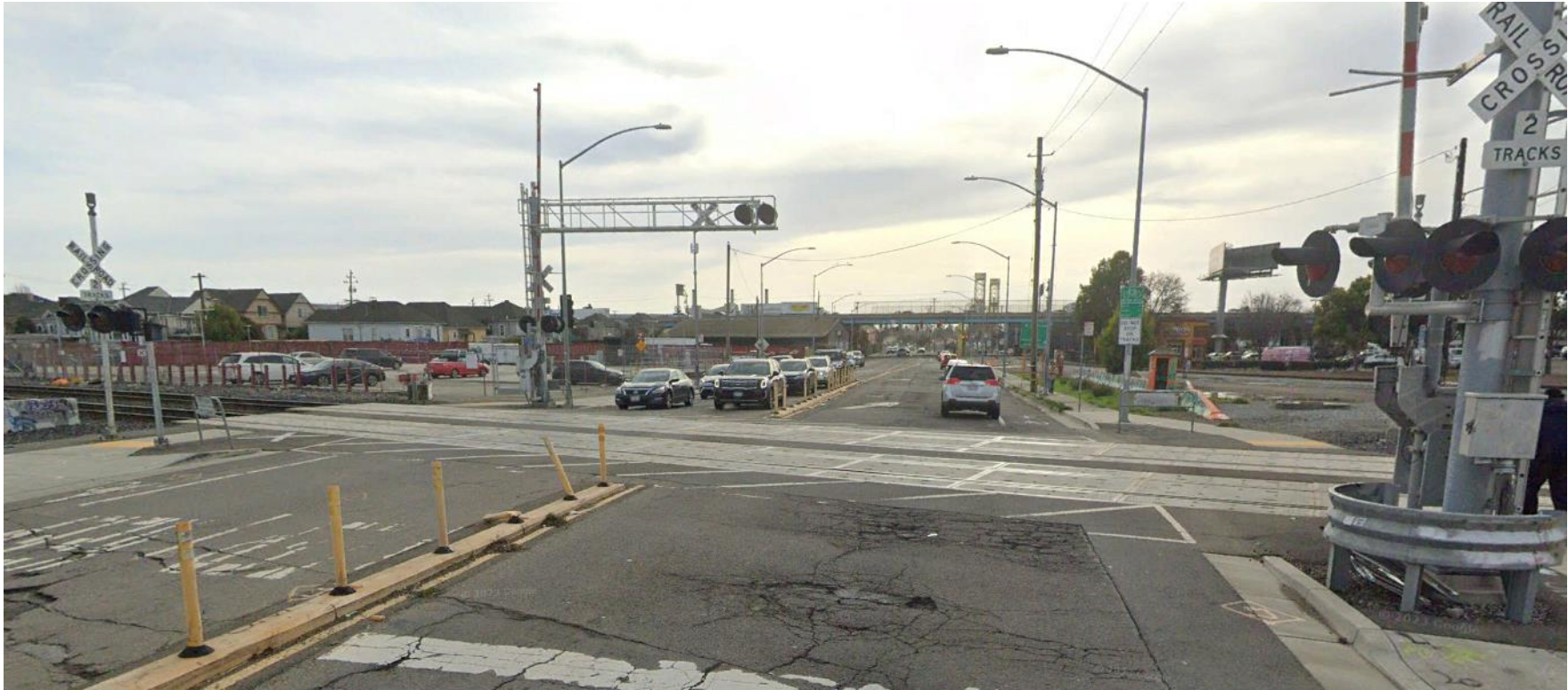
Figure 3: Fruitvale Avenue Crossing
