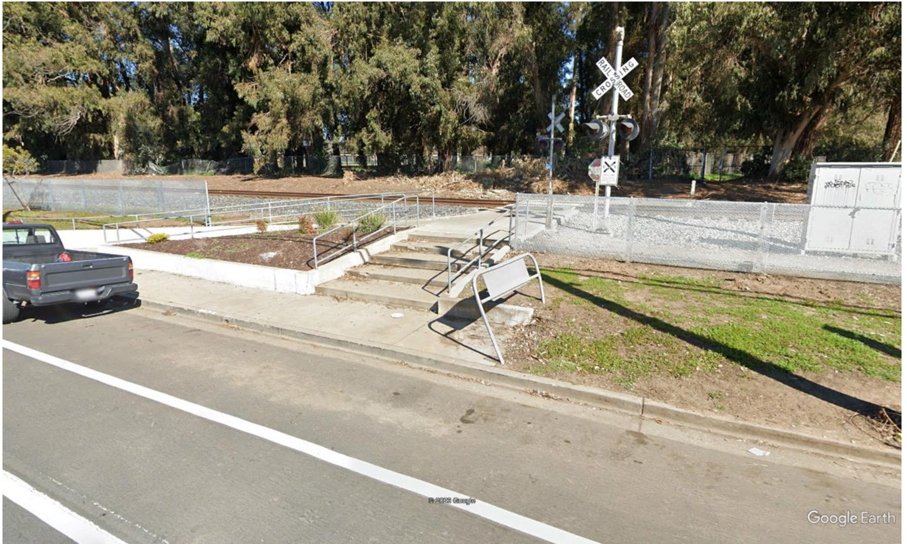
Figure 3-6 Tennyson High School Pedestrian Crossing -Existing Conditions from South looking North
