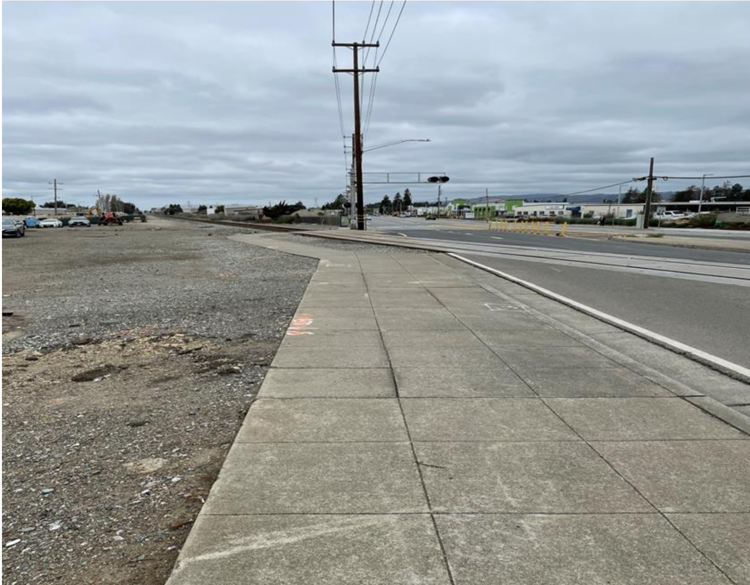
Figure 3-2 Washington Avenue- Existing Conditions from South looking North
