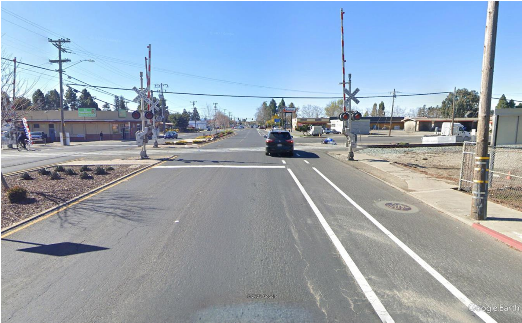
Figure 3-7 Tennyson Road and Leidig Court Trespass -Existing Conditions from Northeast looking Southwest
