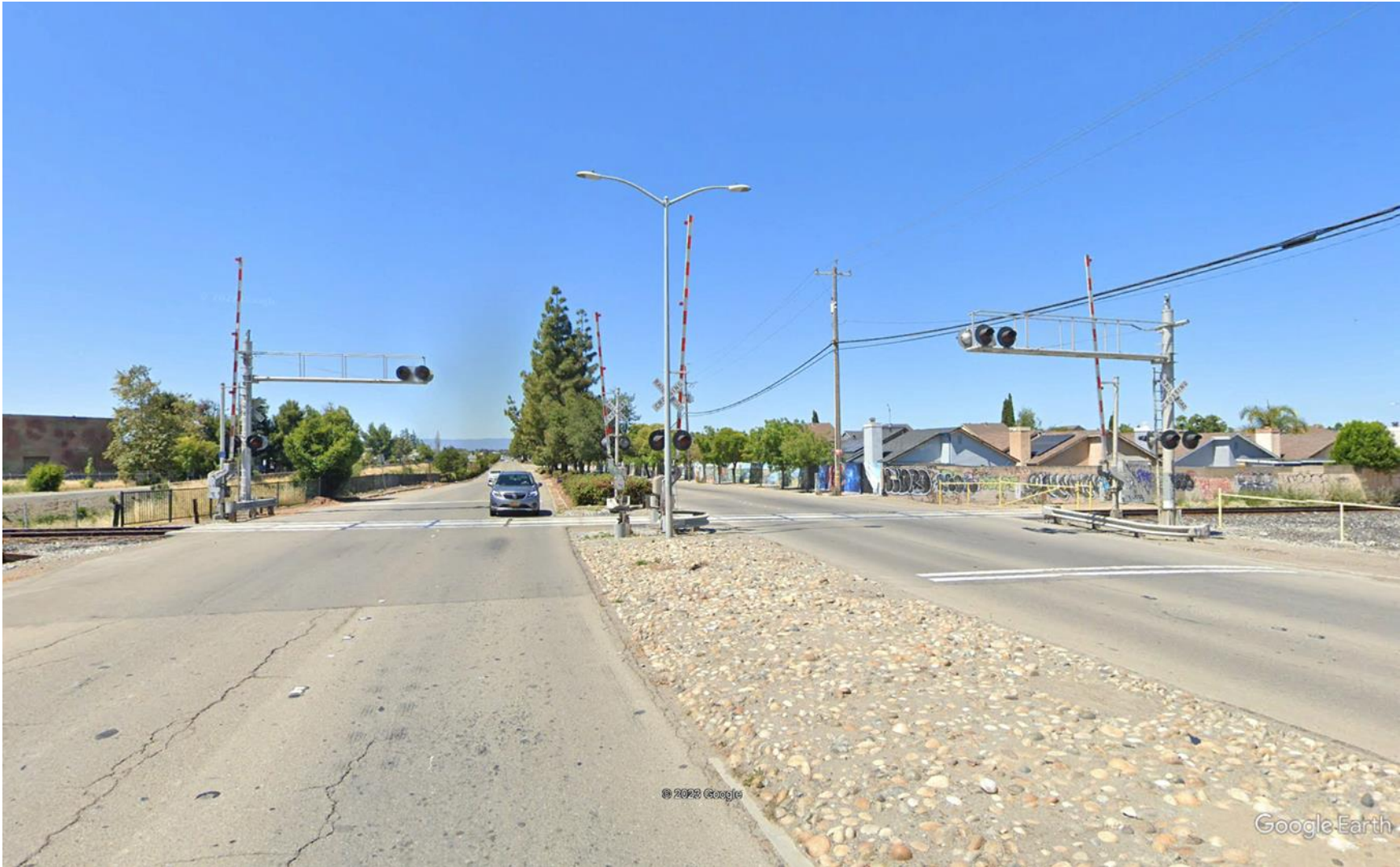
Figure 3-8 Industrial Parkway - Existing Conditions from Northeast looking Southwest
