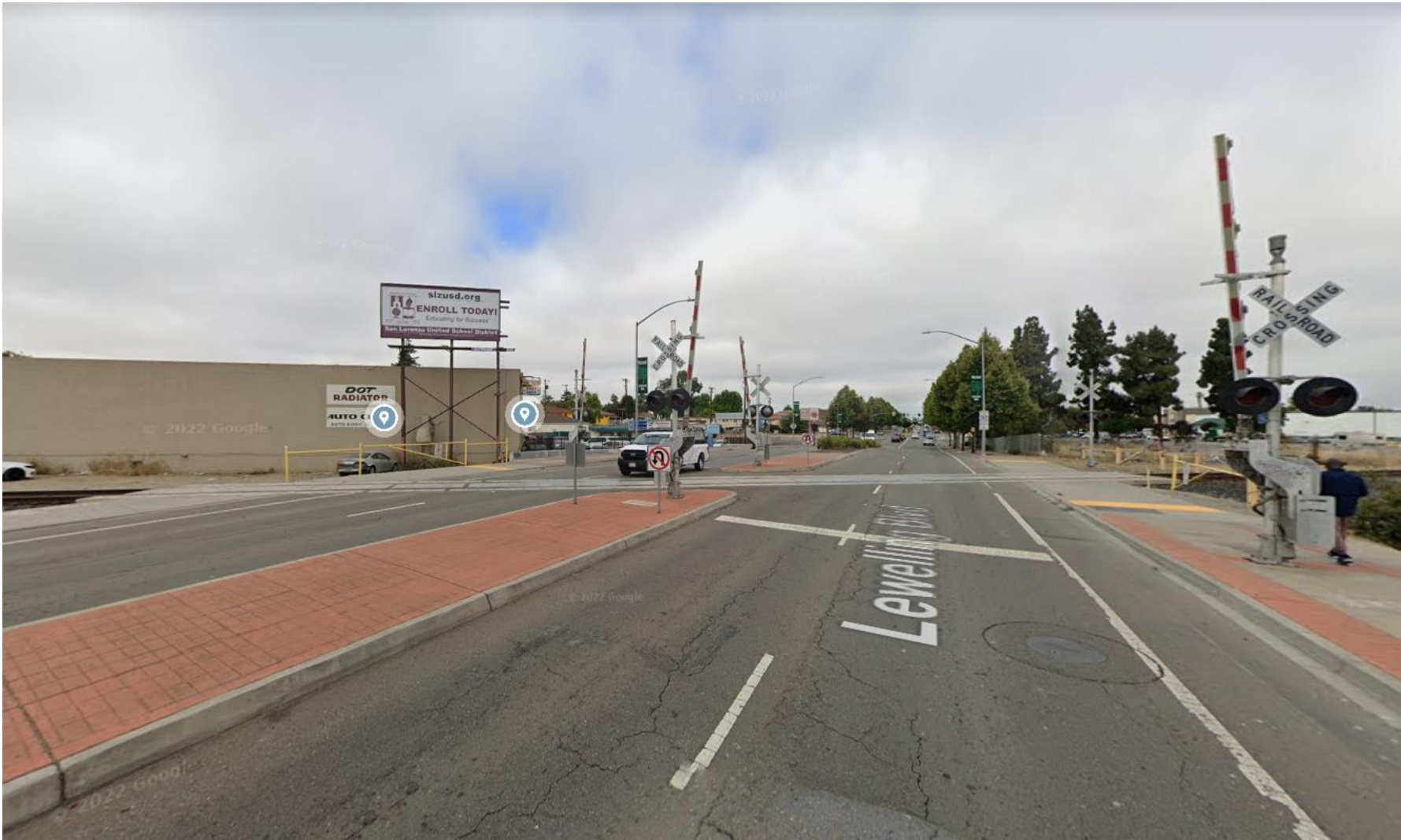
Figure 3-5 Lewelling Boulevard -Existing Conditions from East looking West
