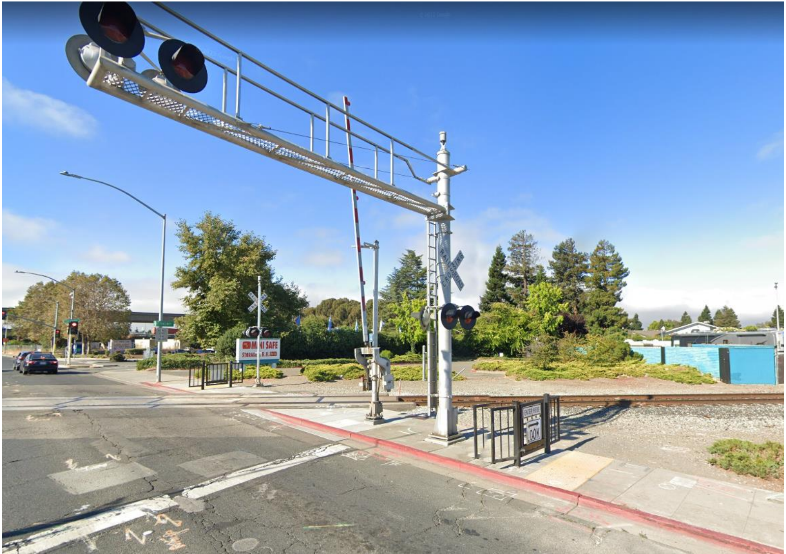
Figure 3-3 Hesperian Boulevard - Existing Conditions from Northeast looking Southwest
