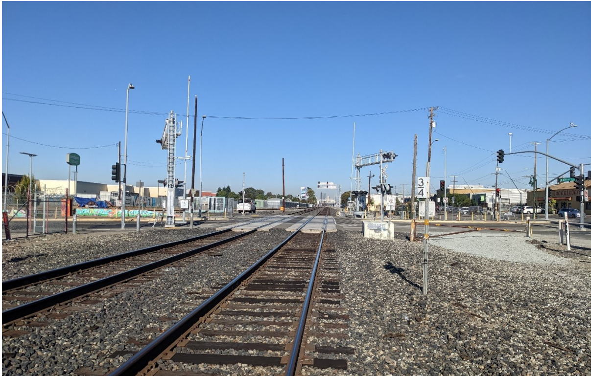
Photograph 7. View of the railroad crossing at Fruitvale Avenue, facing northwest.
