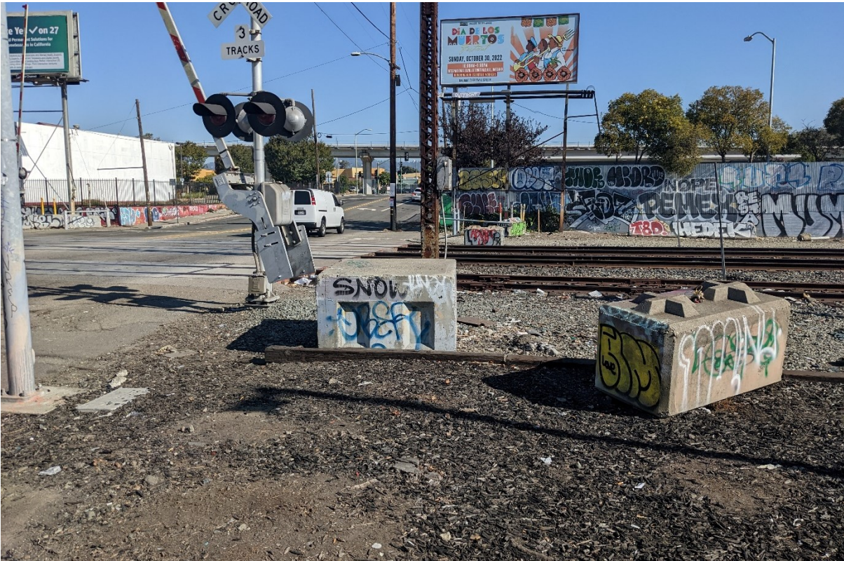
Photograph 2. View of the railroad crossing at 29th Avenue, facing northeast.
