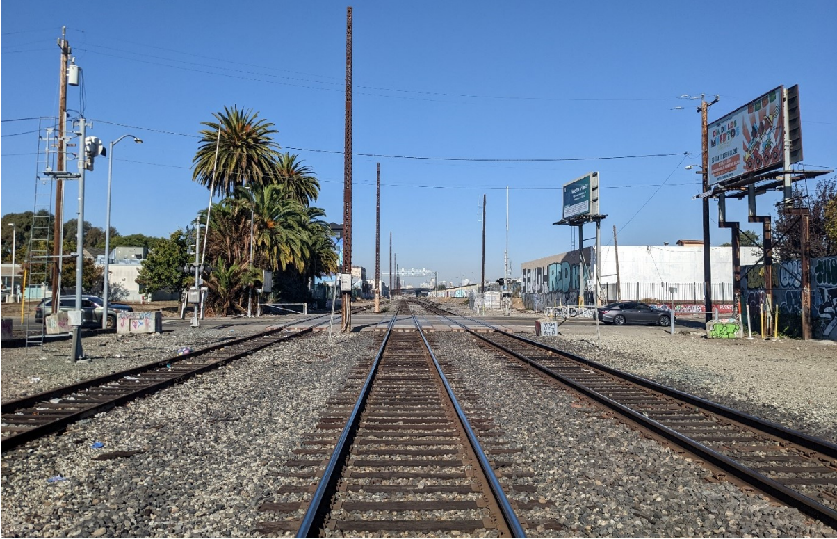
Photograph 1. View of the railroad crossing at 29th Avenue, facing northwest.
