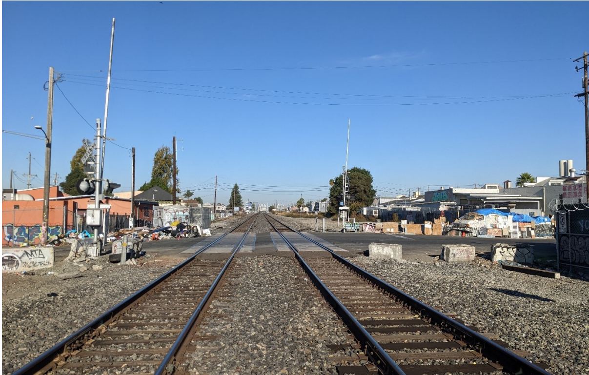
Photograph 3. View of the railroad crossing at 37th Avenue, facing northwest.
