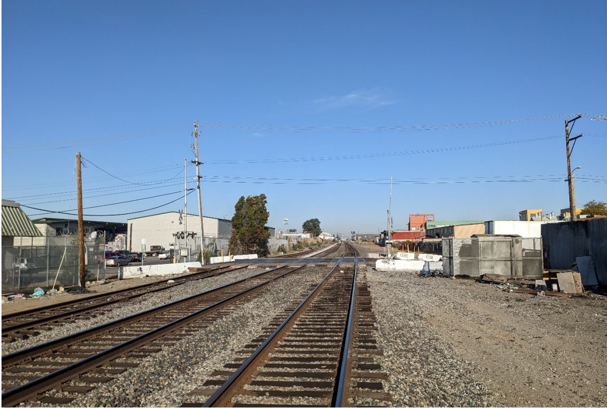
Photograph 5. View of the railroad crossing at 50th Avenue, facing northwest.
