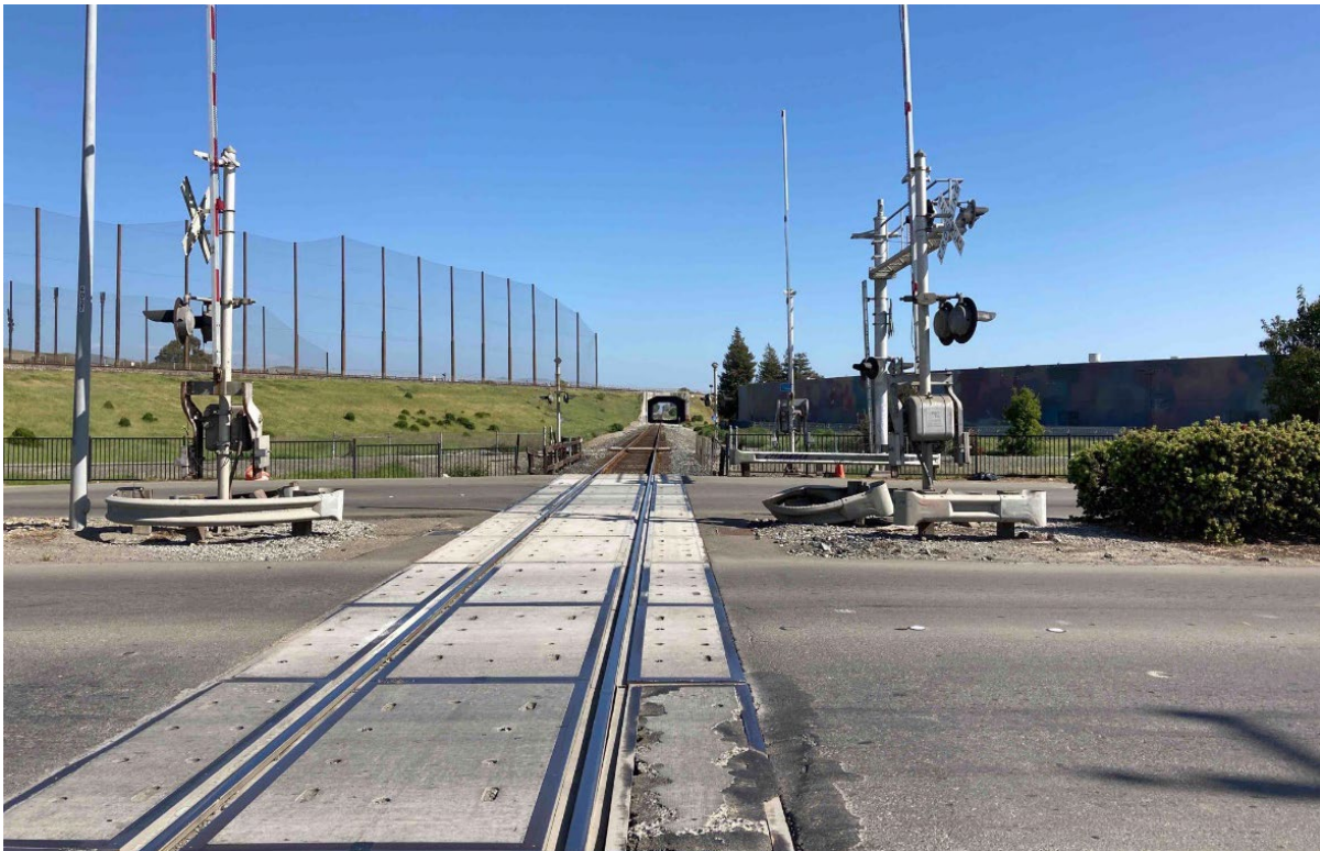
Photograph 362. View of bridge over Ward Creek to the southeast of the Industrial Parkway railroad crossing, facing southeast.
