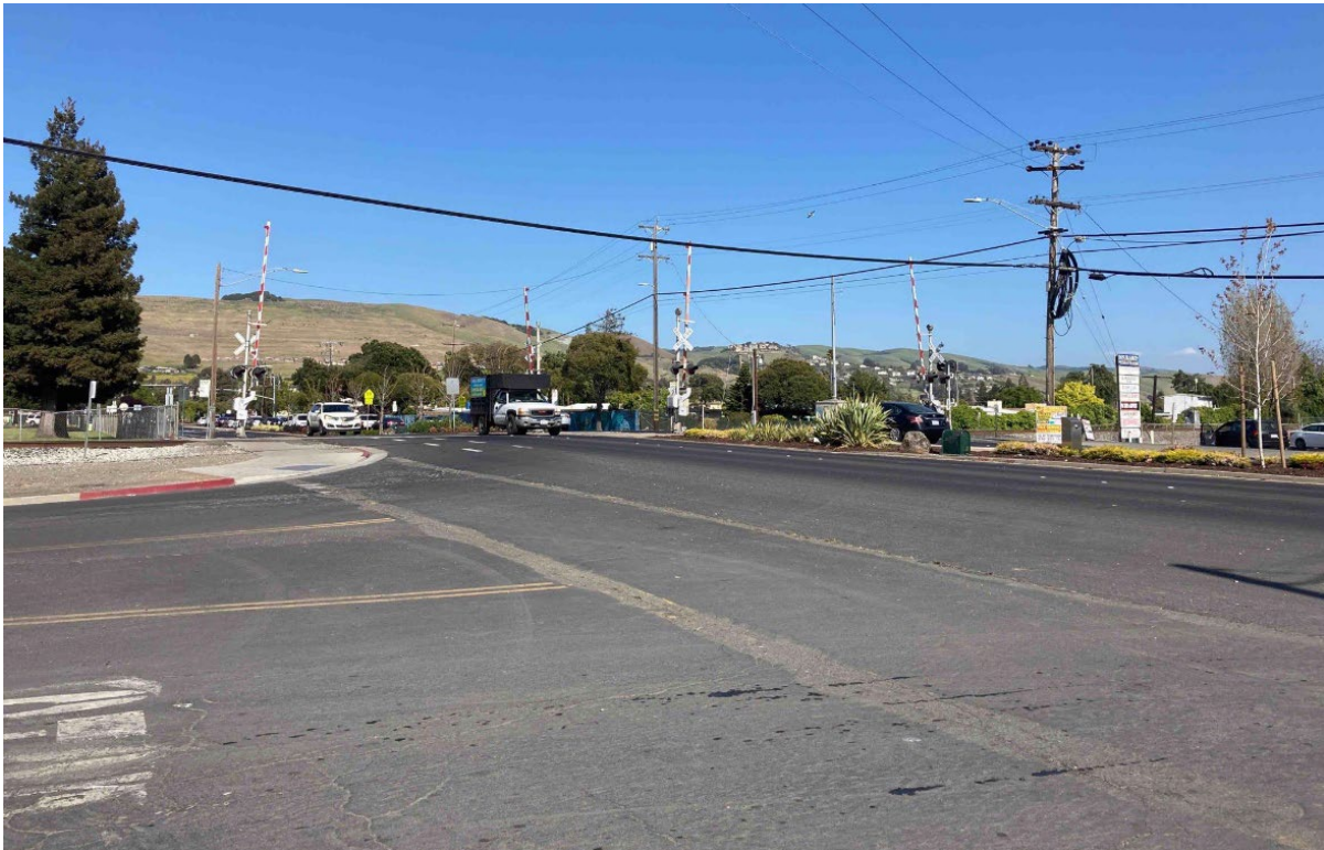
Photograph 24. Overview of the railroad crossing at Tennyson Road, facing east.
