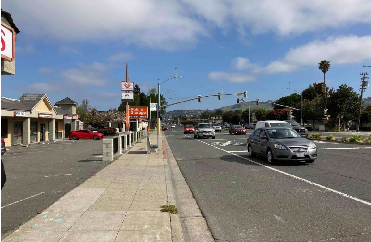
Photograph 10. View of existing pavement marking north of the railroad crossing at Hesperian Boulevard, facing north.
