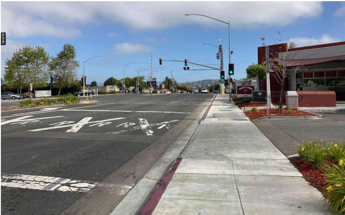
Photograph 12. View of existing pavement marking south of the railroad crossing at Hesperian Boulevard, facing north.
