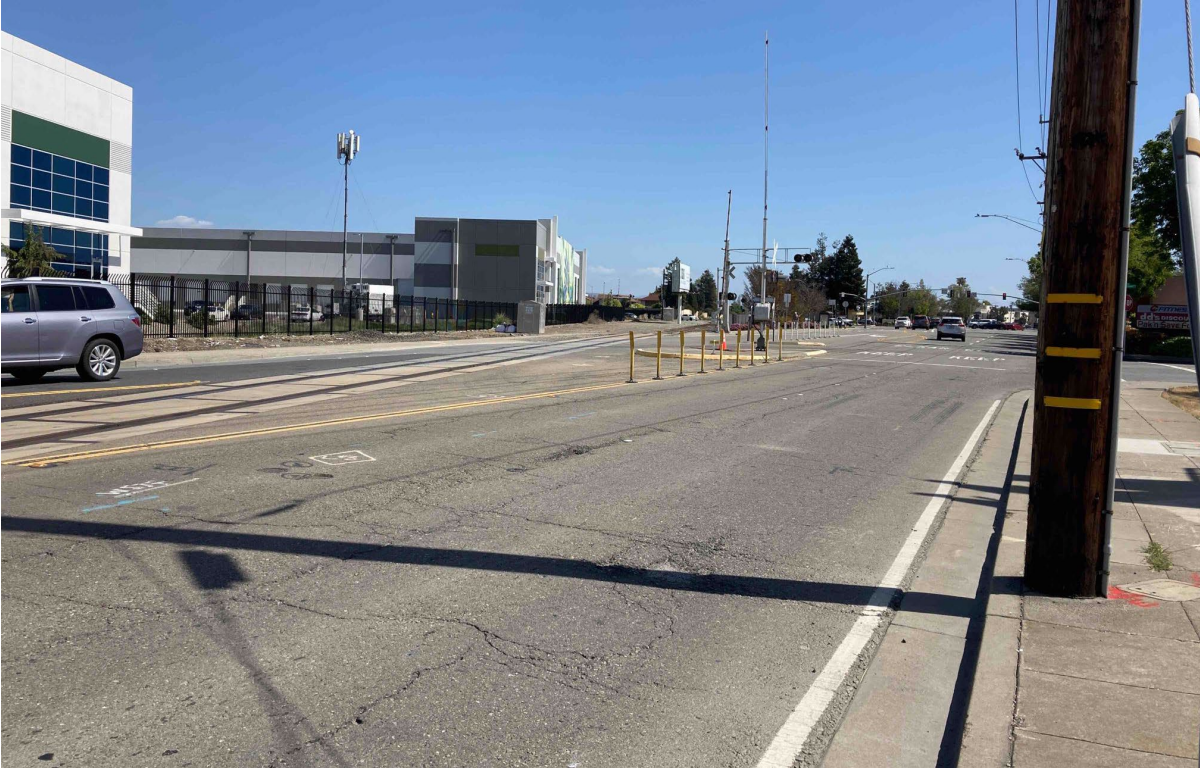
Photograph 6. View of railroad crossing at Washington Avenue, facing southeast.
