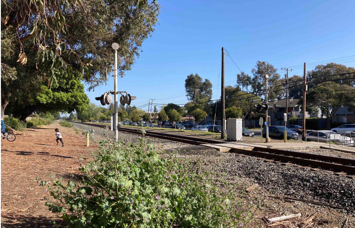
Photograph 21. View of Tennyson High School pedestrian crossing, facing south-southeast. Leidig Trespass Area extends to the south along Huntwood Avenue.
