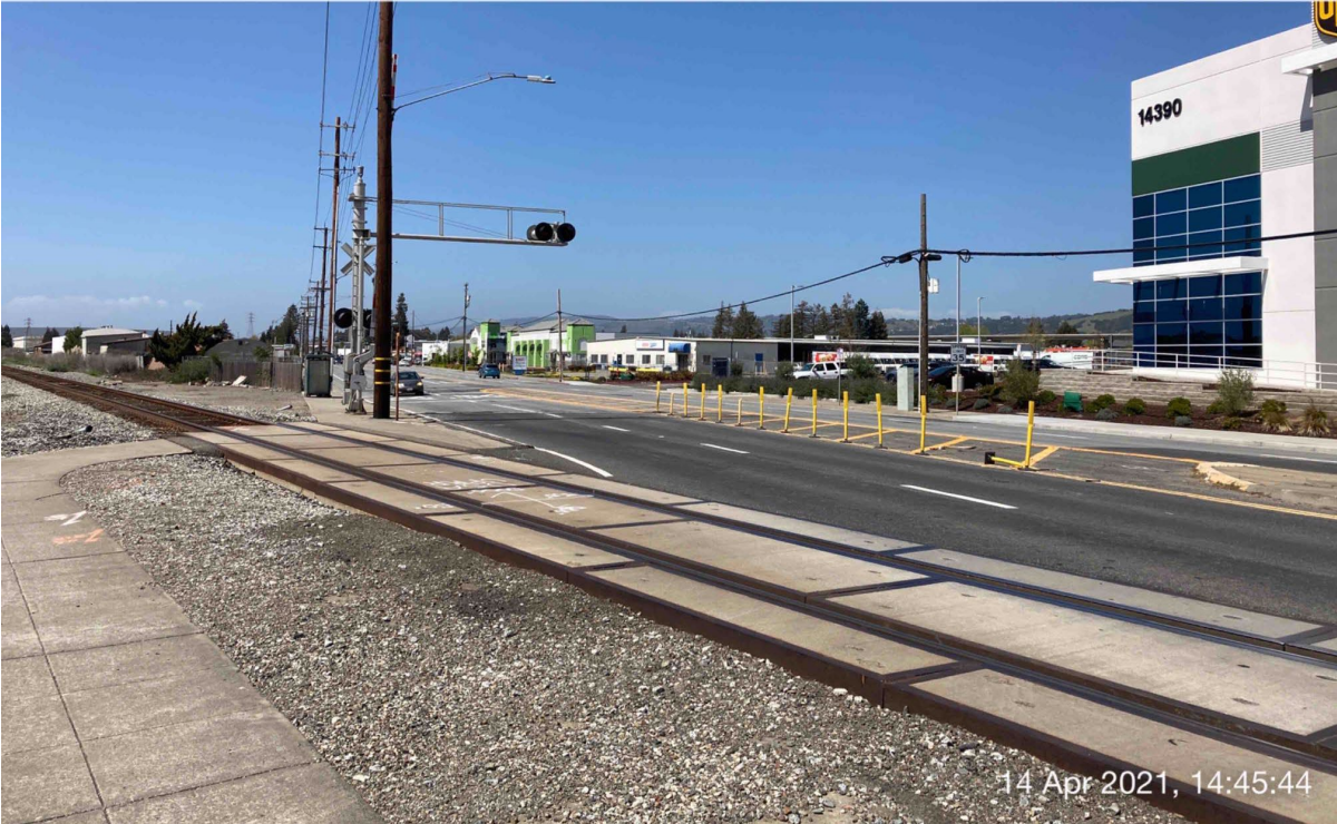
Photograph 5. View of existing pedestrian crossing at Washington Avenue railroad crossing, facing north.
