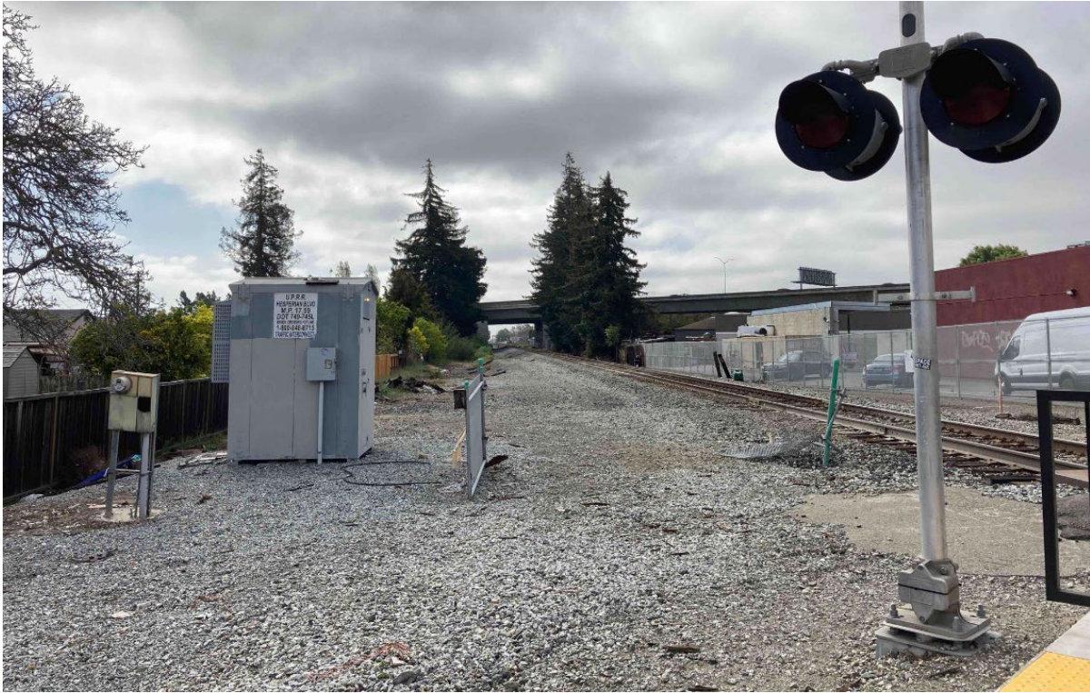
Photograph 11. View of railroad tracks east of existing pedestrian crossing on the north side of the Hesperian Boulevard crossing, facing southeast.
