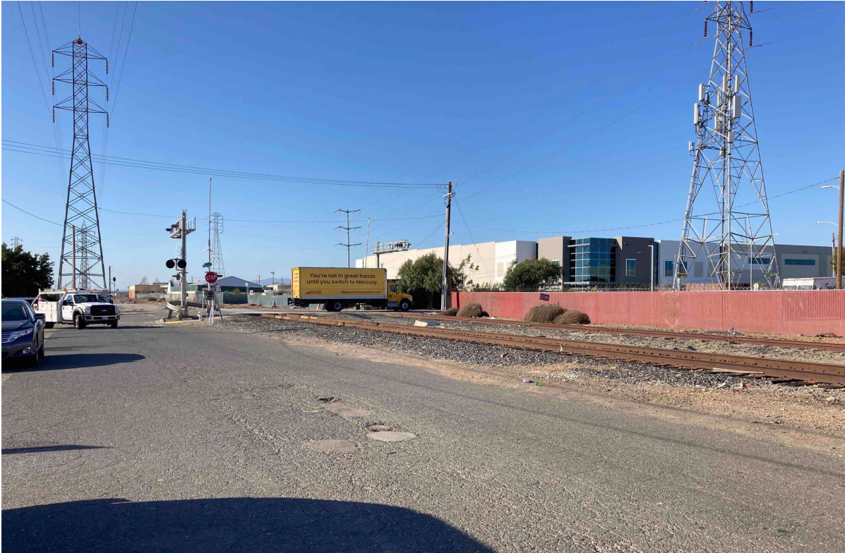
Photograph 2. View of the railroad crossing at Marina Boulevard (coast) from the south, facing north.
