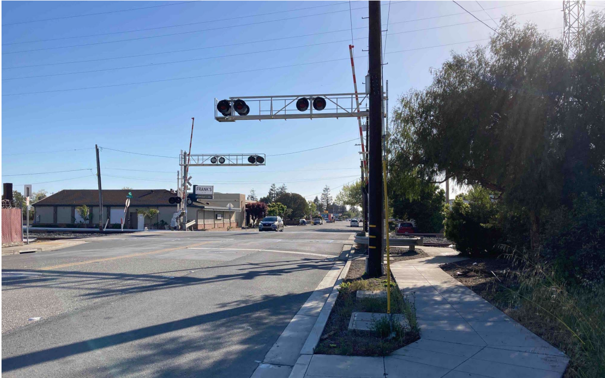
Photograph 3. Overview of the railroad crossing at Marina Boulevard (Coast) from the northeast corner, facing southwest.
