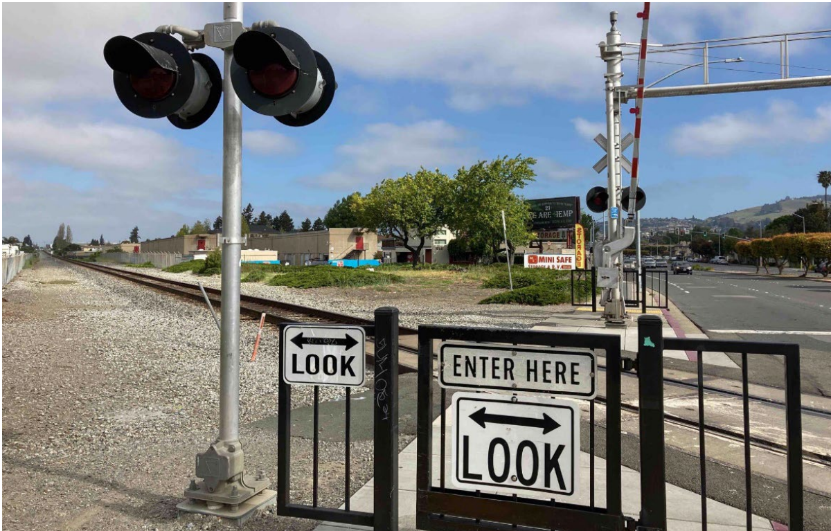
Photograph 8. View of existing pedestrian crossing on the west side of the Hesperian Boulevard railroad crossing, facing north.
