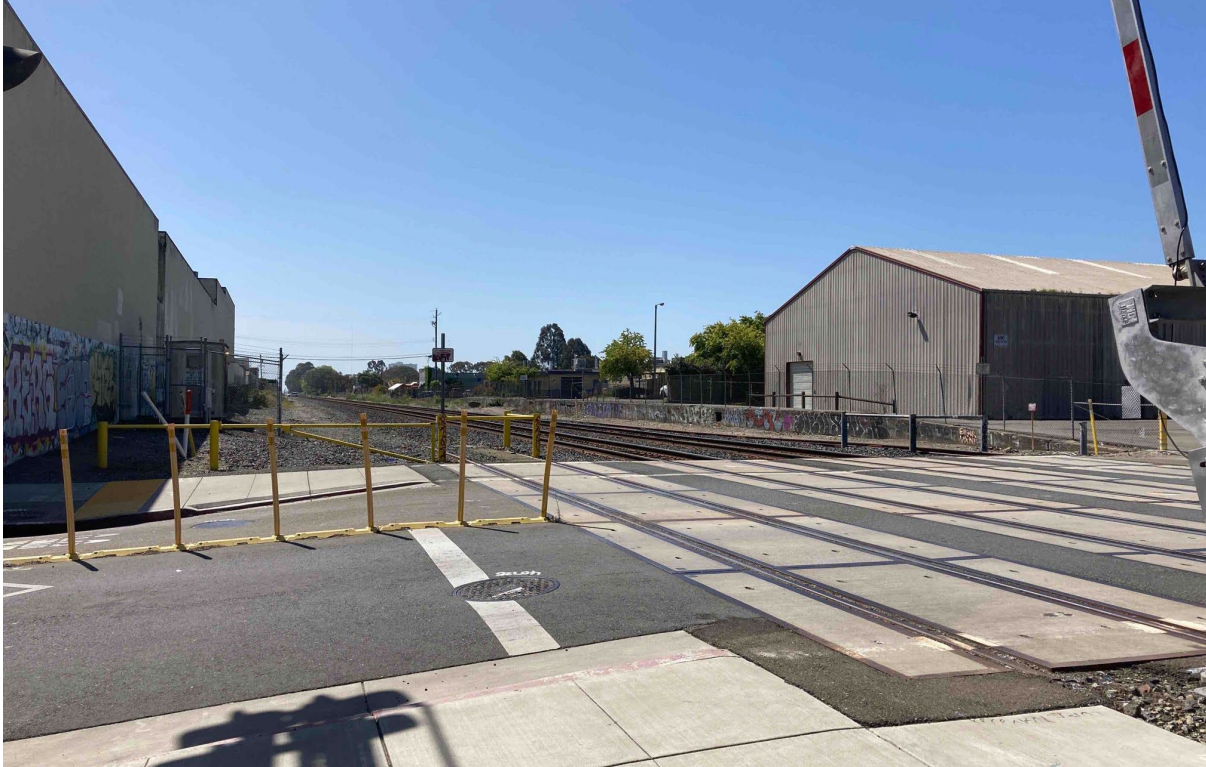
Photograph 7. View of the railroad crossing at Addison Street, facing south.
