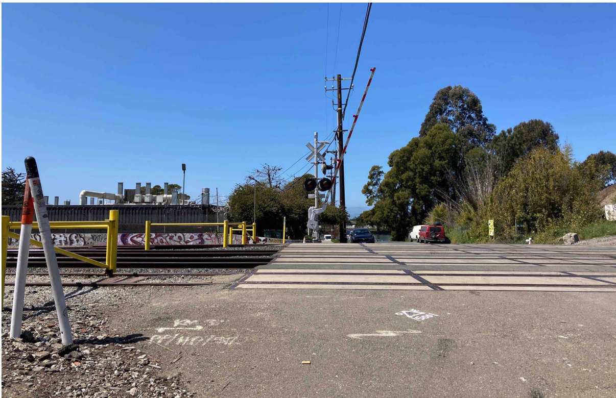
Photograph 10. View of the railroad crossing at Bancroft Way, facing west.
