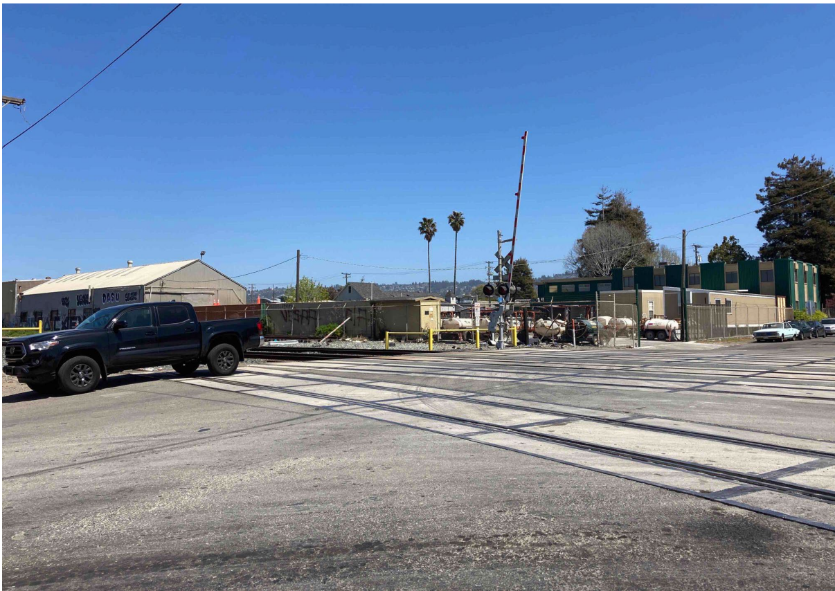
Photograph 4. View of the railroad crossing at Cedar Street, facing northeast.
