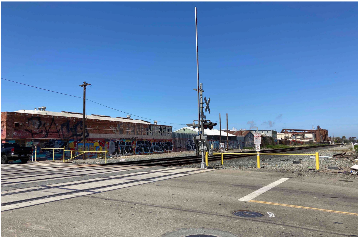
Photograph 2. View of the railroad crossing at Cedar Street, facing northwest.
