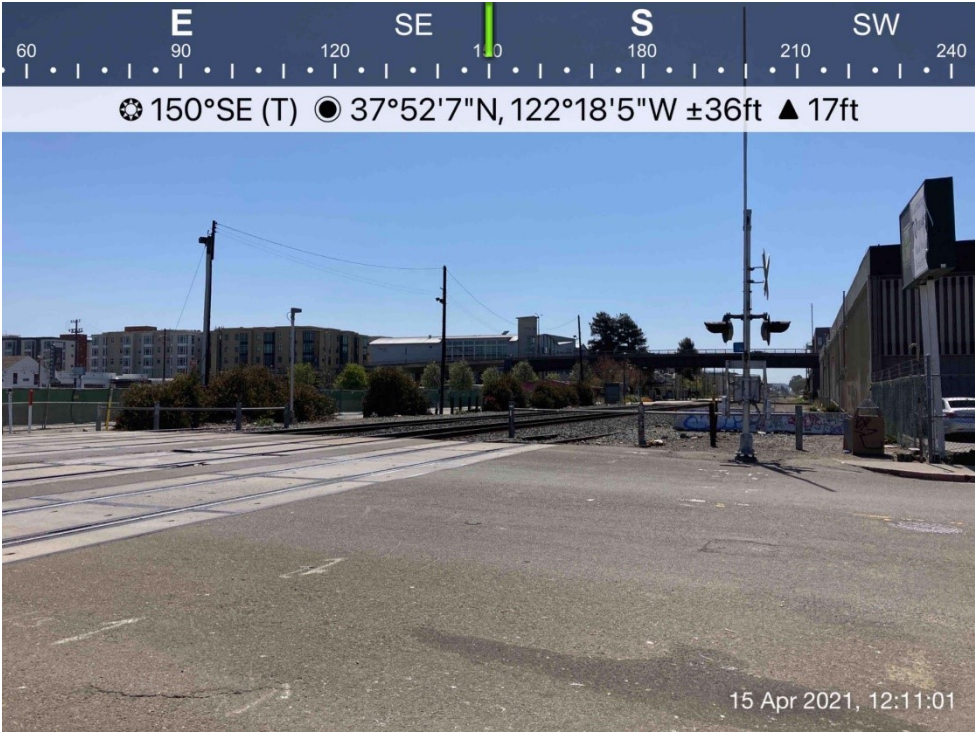
Photograph 4. Hearst Avenue, Berkeley - overview of railroad crossing from northwest corner, facing southeast.
