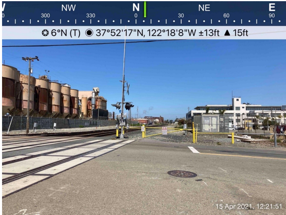
Photograph 1. Virginia Street, Berkeley - overview of railroad crossing from southeast corner, facing north.
