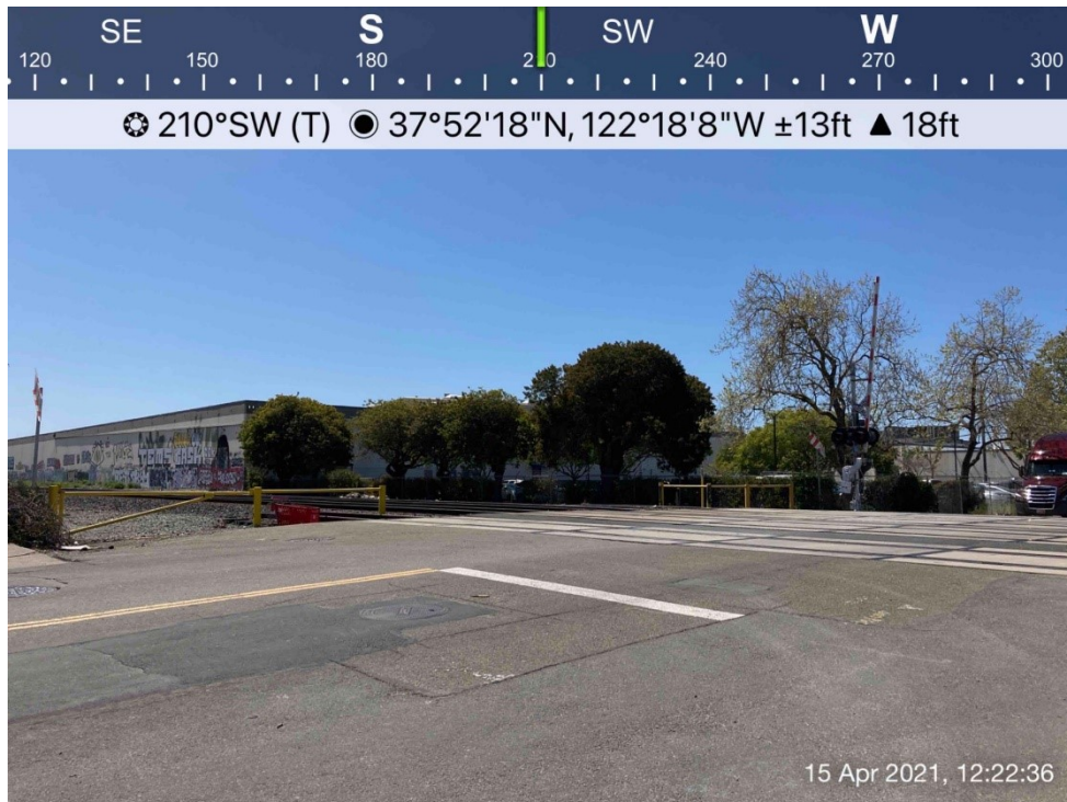
Photograph 2. Virginia Street, Berkeley - overview of railroad crossing from northeast corner, facing southwest.
