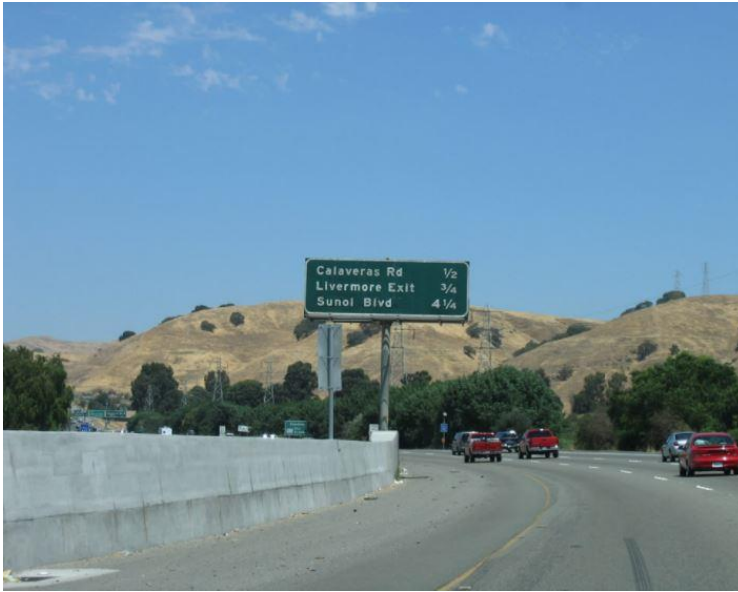
I-680 northbound approaching the Calaveras Road off-ramp.
