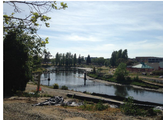
Figure 3-5. Lake Merritt Channel
