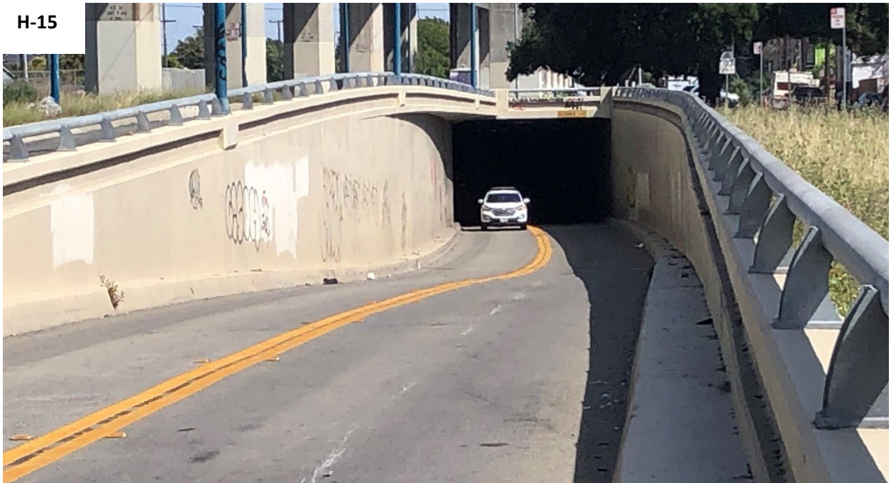
H-14-15 | San Leandro Street Underpass at 105 th Avenue in Oakland: There is a lack of signage to warn pedestrians and cyclists of unsafe road conditions, and no direct route southbound on San Leandro Street
