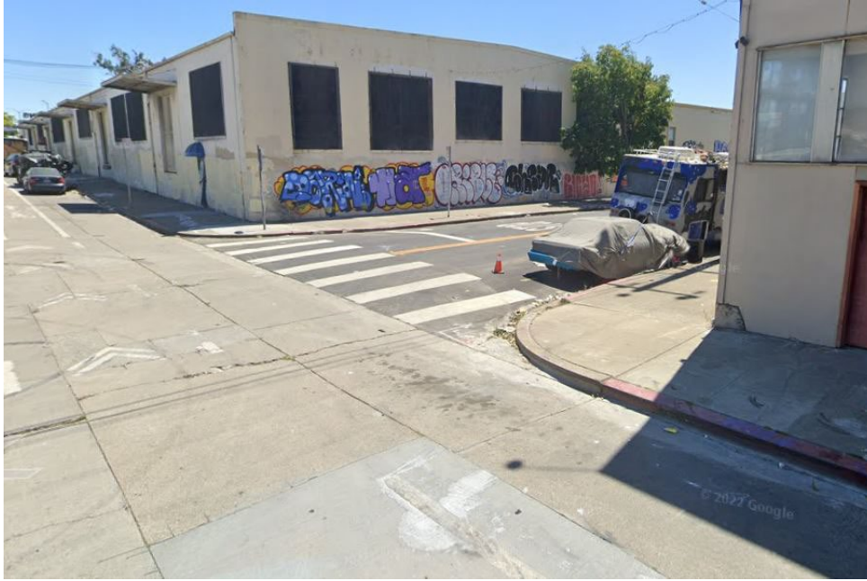
H-3 | E10 th Street at 8 th Avenue in Oakland: Several blocks on E10 th Street have no curb ramps or are otherwise not ADA compliant
