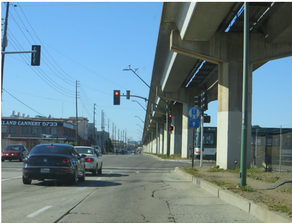
H-8 | E12 th Street at 25 th Avenue in Oakland: Unprotected left turns on E12 th Street are aggravated by poor sight distance due to the presence of the BART aerial structure columns
