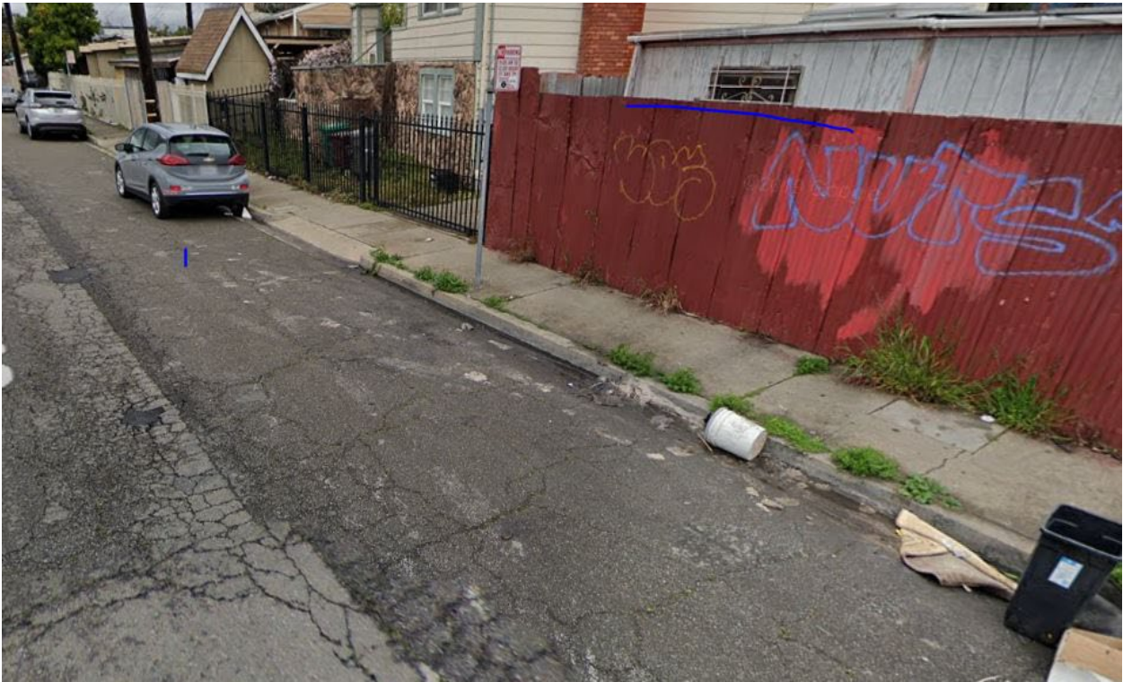
H-19 | San Leandro Street at Blenheim Street in Oakland: Pedestrians and cyclists must contend with narrow sidewalks and poor pavement conditions
