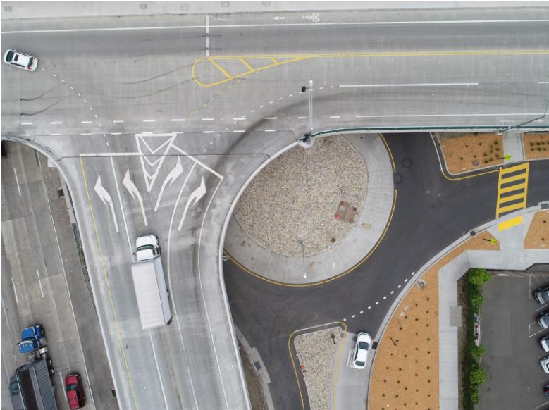
Aerial view of the 29th Avenue off-ramp and roundabout.
