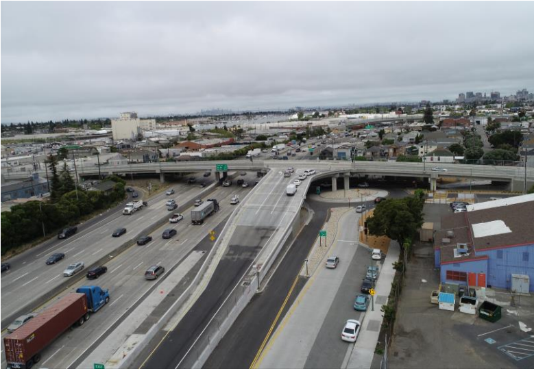
29th Avenue off-ramp and roundabout and overcrossing structure.
