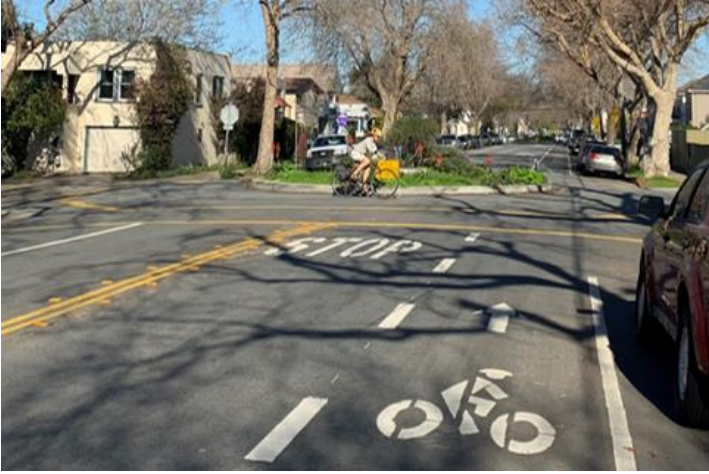
Existing bike boulevard route showing roundabout and crossing treatment.
