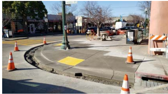
City of Albany – Lower Solano Curb Ramp Improvements
