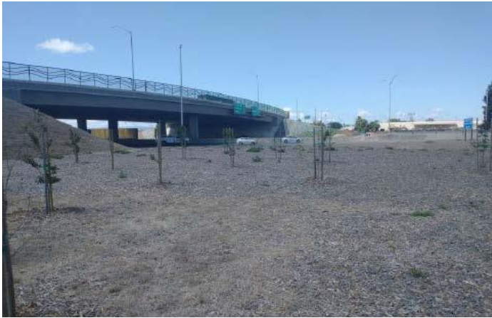
I-880 and Marina Boulevard Overcrossing – First Year of Plant Establishment Period.
