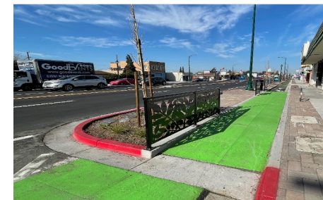
Protektadong daanan ng bisikleta na may green stormwater infrastructure buffer (Phil Erickson, CD+A)
