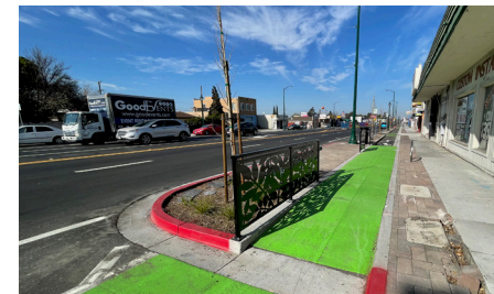
A bus island and protected bikeway along Adeline Street in Berkeley, CA. (Amanda Leahy / Kittelson & Associates, Inc.)
