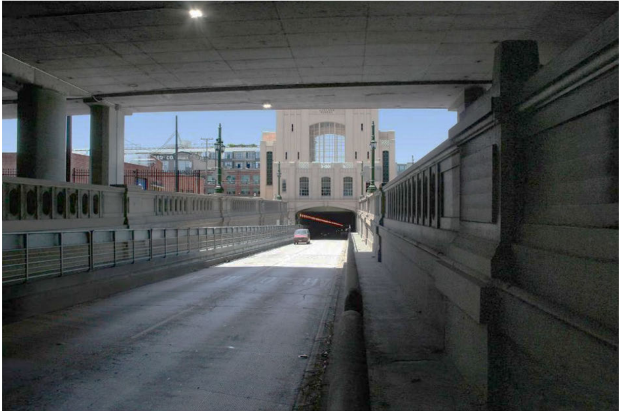
Source: Visual Impact Assessment (VIA) (April 2020)
