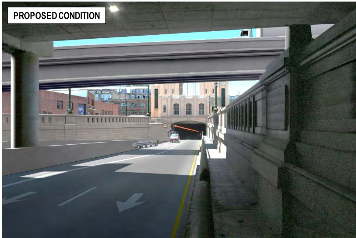
Figure 2-24. Viewpoint 5 on Harrison Street Looking South at the Posey Tube
