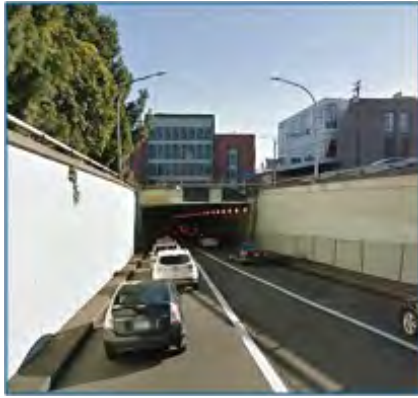
Existing view of entrance to the Webster Tube.
