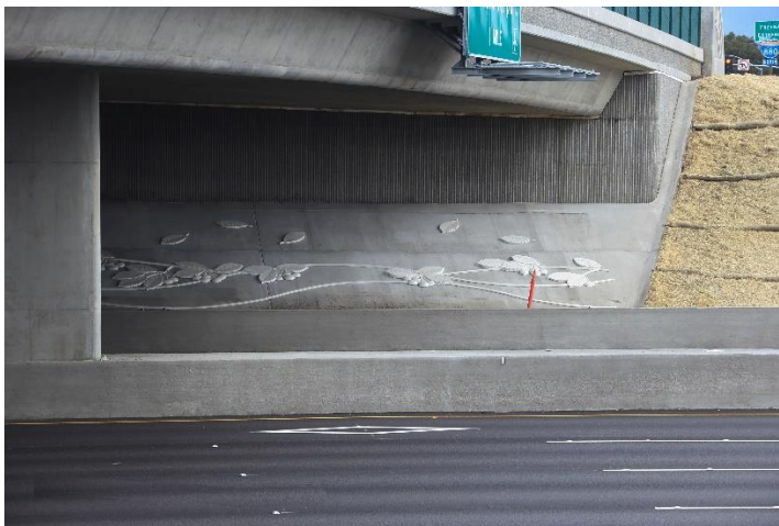
Decorative slope paving along Interstate 880, Courtesy of the California Department of Transportation
