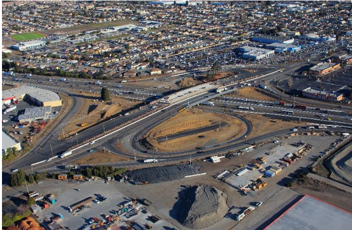
Aerial photograph of Interstate 880/Davis Street interchange, Courtesy of the California Department of Transportation
