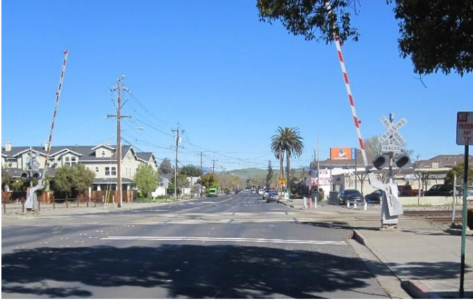
A typical at-grade crossing that requires improvement. This location is at L Street in the City of Livermore.
