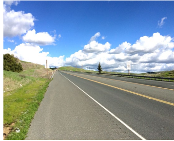
SR-84 looking westbound near Ruby Hill Road.
