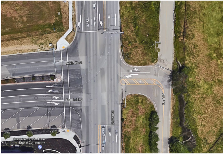
Beginning of road extension at Dublin and Fallon intersection.
