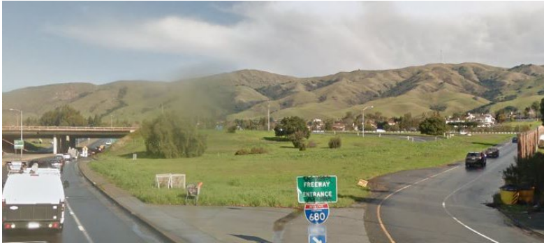
Eastbound SR-262 at the I-680 southbound on-ramp.
