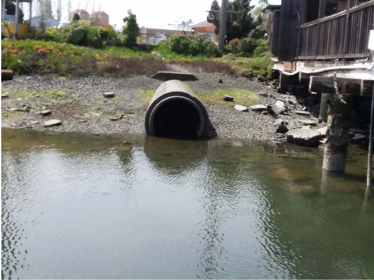
13) Photograph of 45" concrete culvert at Barnhill Marina, looking south.
