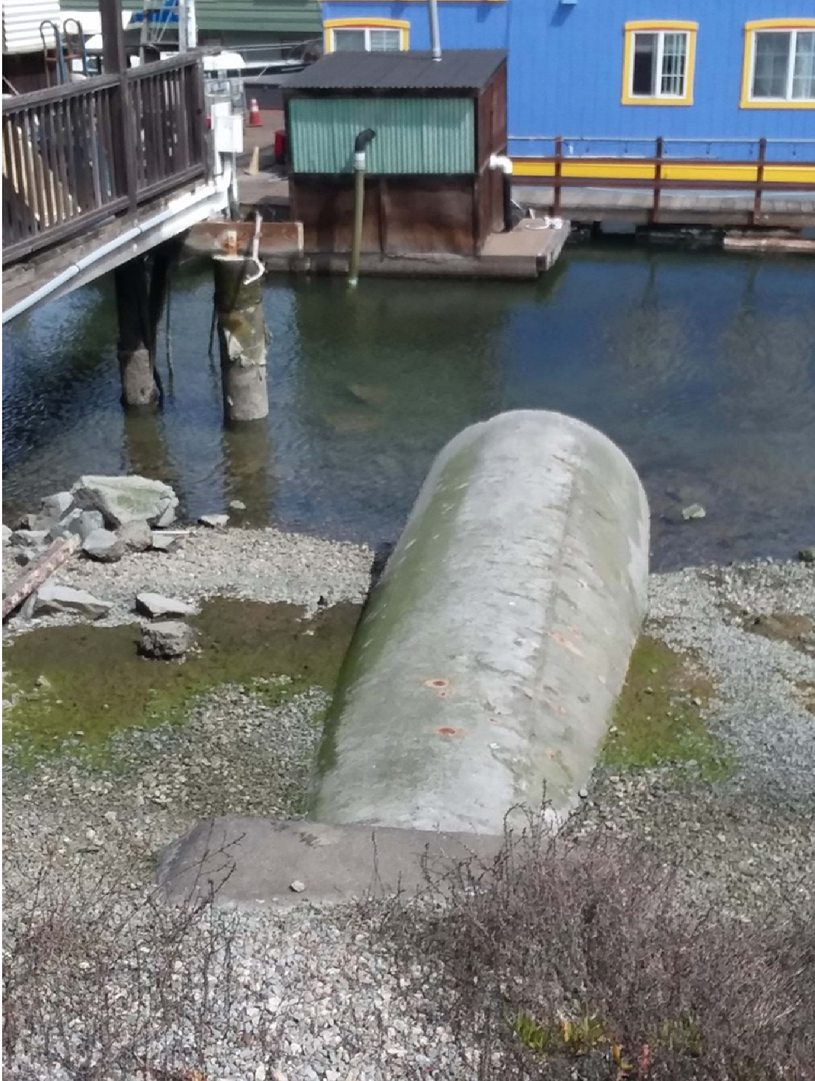
12) Photograph of 45" concrete culvert outfall at Barnhill Marina, looking north.
