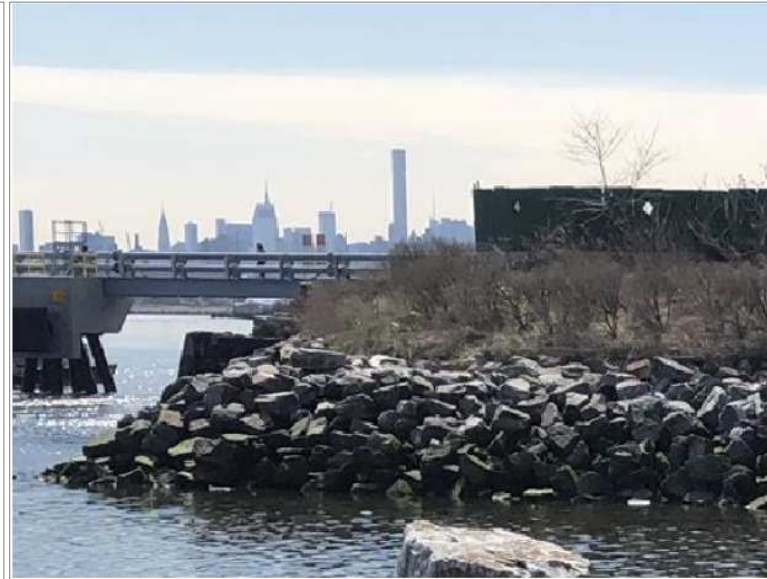
Photo 4-4: Rubble mound structure in Bronx, New York (M&N, 2017)
