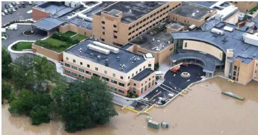
Photo 4-5: Flip-up barrier at Lourdes Hospital deployed automatically during a recent flood event (Floodbreak)
