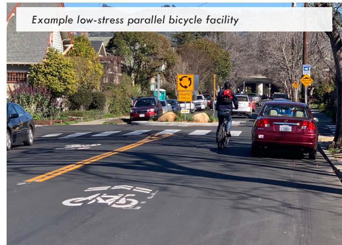
Figure 13: Shafter Avenue Bicycle Sharrows & Roundabout, Oakland
