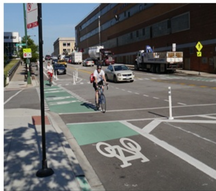
(B. Protected intersection, example picture only)
