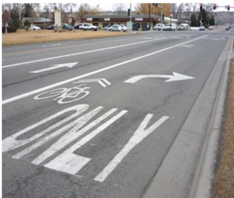
(A. Bike facility mixing with other traffic at intersection, example picture only)
