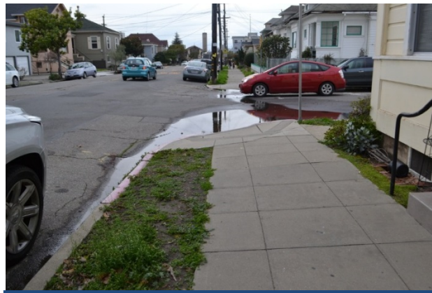
Essex and Alcatraz (needs marked crosswalk)
