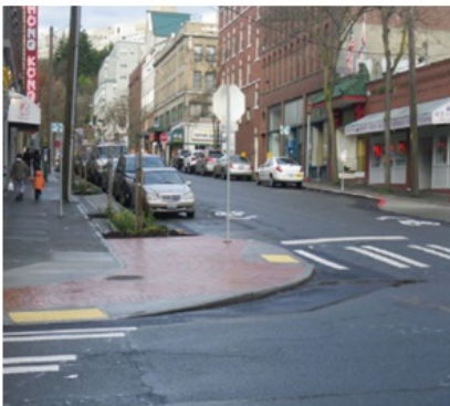
(A. An extension of the curb to shorten crossing distances at intersections on San Pablo Avenue, with bike facilities on parallel streets.)
