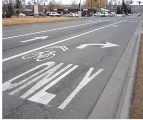
(B: Bike facility mixing with other traffic at intersection, example picture only)
