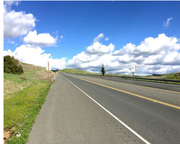
SR-84 looking westbound near Ruby Hill Road.
