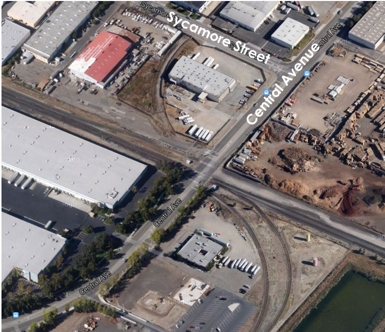
Central Avenue near Sycamore Street.
